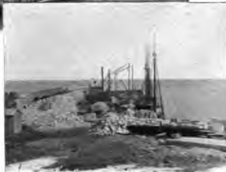
PIGEON HILL GRANITE COMPANY'S PIER.
